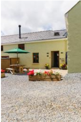
Main Entrance to the Barn
